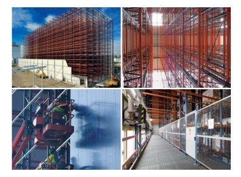
The warehouse is built with 10 cm thick sandwich panels and include a polyurethane (PUR) insulation core
